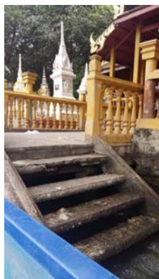
Fig. 10 The steep ladder pier
