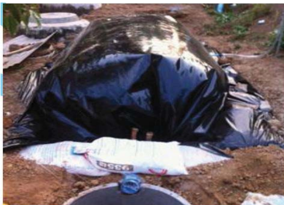
Fig. 6 Test the digester of biogas system
