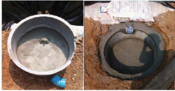
Fig. 5 Prepare pothole of fill dung
